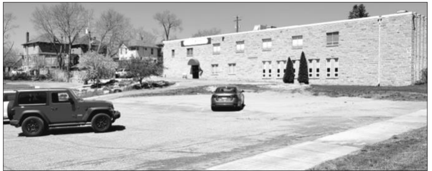
History Center Parking Lot April 26, 2024
