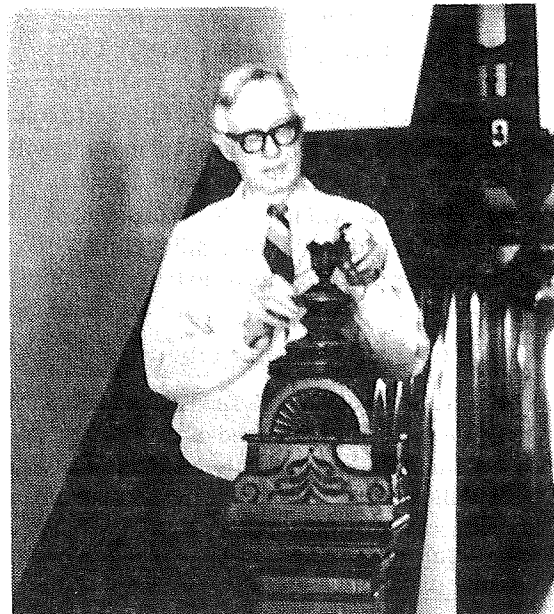
Dr. Larry Hammer demonstrates measuring to duplicate wood carvings on a newell post
