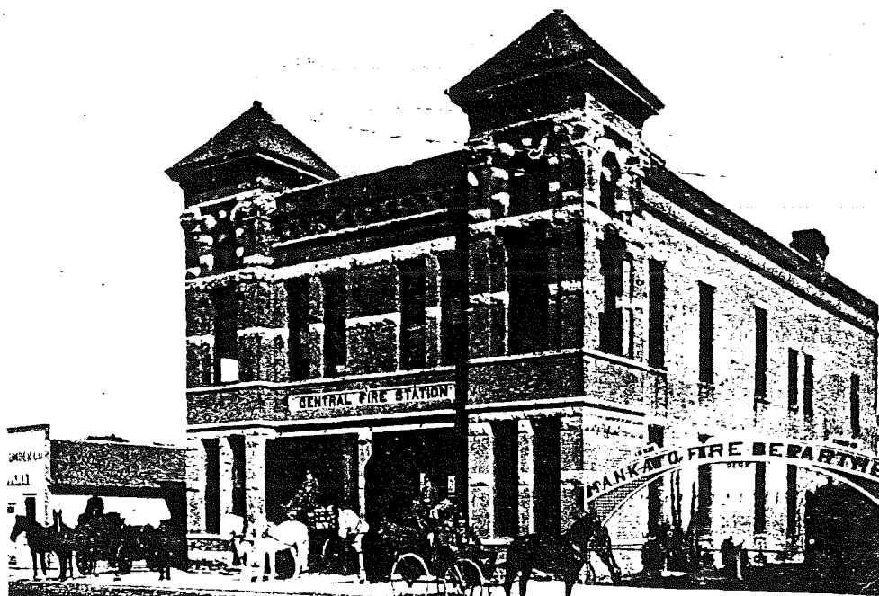
Central Fire Station, 121 S. Second St., Mankato -- (BECHS Collection)
