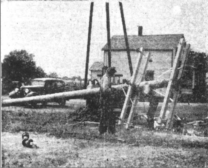
Installation of some of the first electric poles. Mankato Free Press , July 2, 1938
