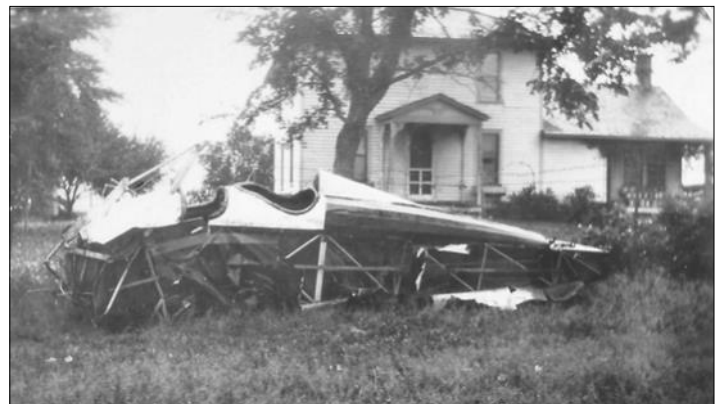
The plane after it had been removed from the school roof.
