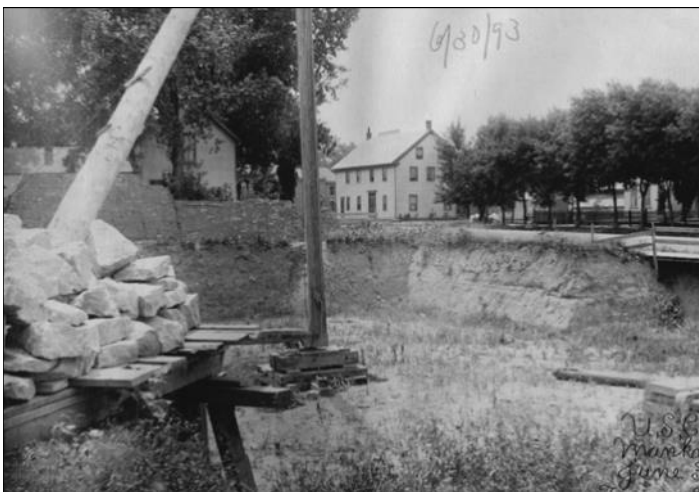
Excavation and construction, June 30, 1893.
