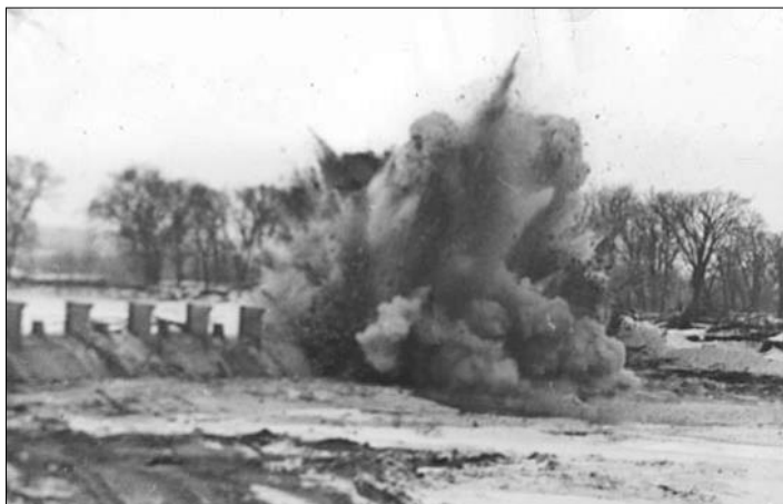
Dynamiting the dam, January 1952
