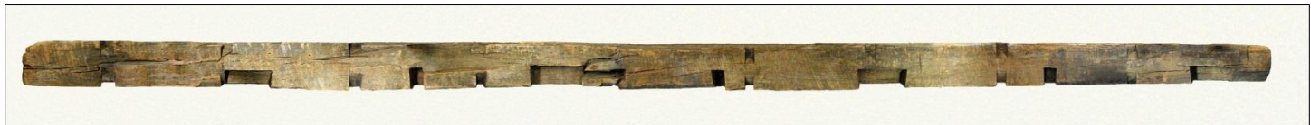
Entire timber view, Floor Sill "This Side Up"
